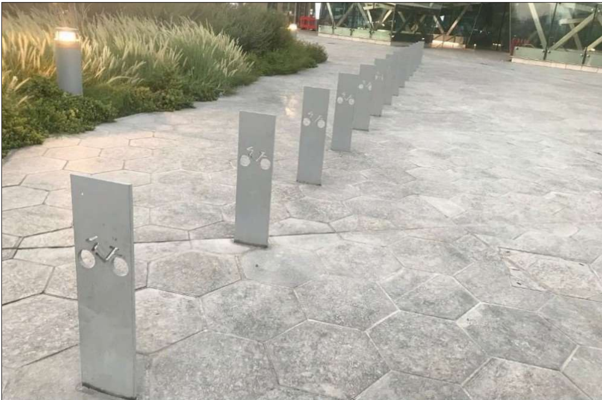
Figure 13-7 Wide Post Rack Bicycle Parking (Msheireb Metro Station)
